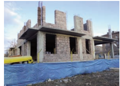
The second floor near completion
